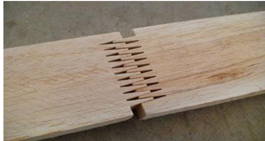
Figure 1: A finger jointed timber section
