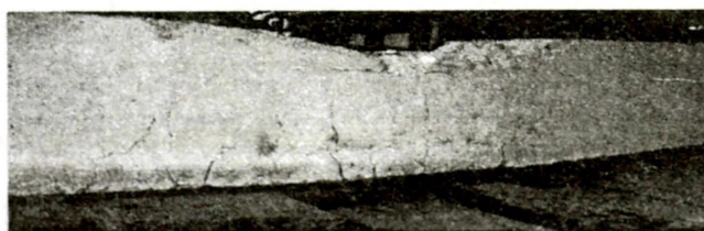
Figure 12: Cracks locations of 1% of bamboo + 1% of steel with steel stirrups
