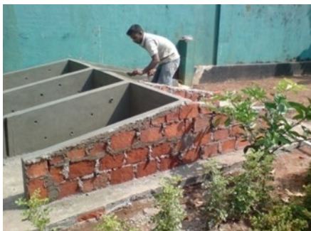
Figure 2: SBCs are being constructed
