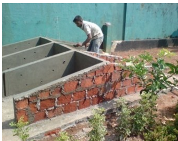
Figure 2: SBCs are being constructed
